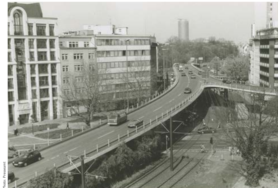
◀ Built in 1962, demolished in 2013: The ‘Tausendfüßler’ flyover
