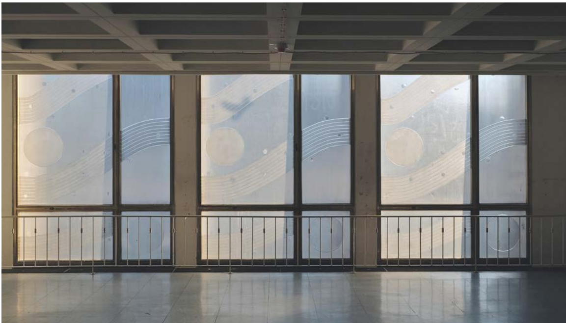
Ewald Mataré, Düsseldorf-Pempelfort, former Düsseldorf North tax authority office, glass wall on the upper floor
